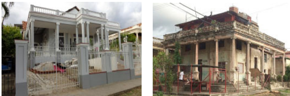
Figure 4: Private initiative to recover a former house to host a bar (left). Example of all issues referred to in one building (right), i.e., deterioration and adverse transformations due to several subdivisions and occupation of front garden for an informal cafeteria. Photographs: Blanc, 2018; Vilorio, 2017
